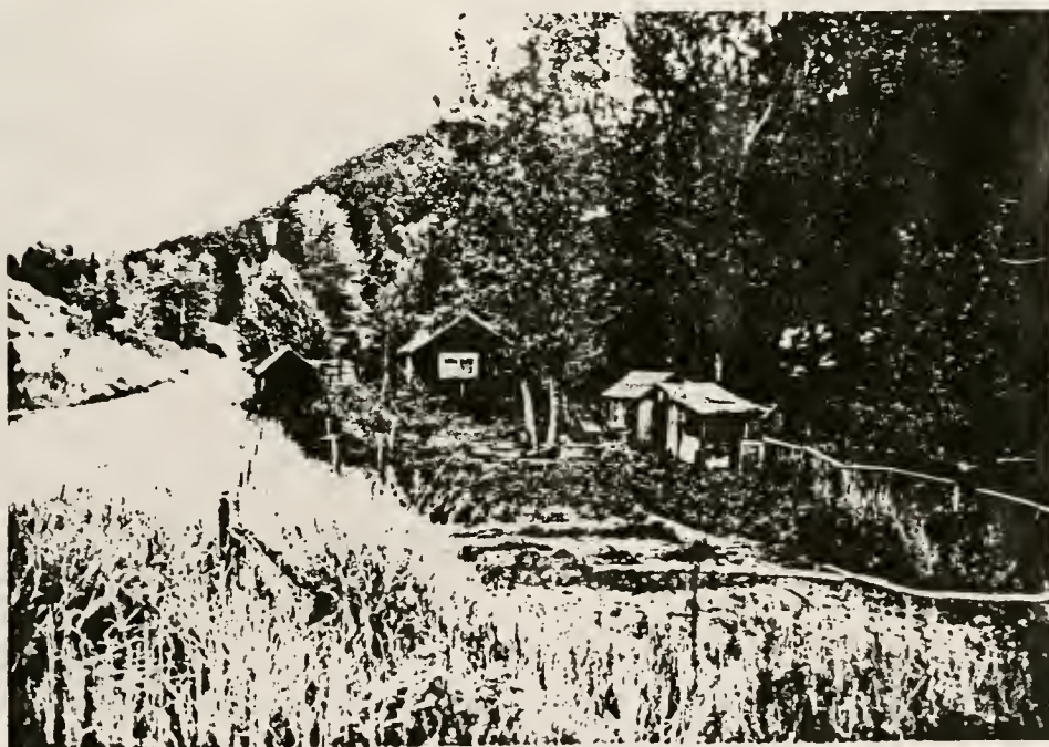
Figure 55. Structure Complex #12, north view.
